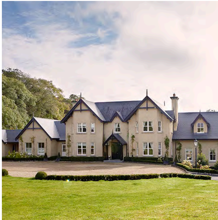
Front elevation where scaffold will be erected
